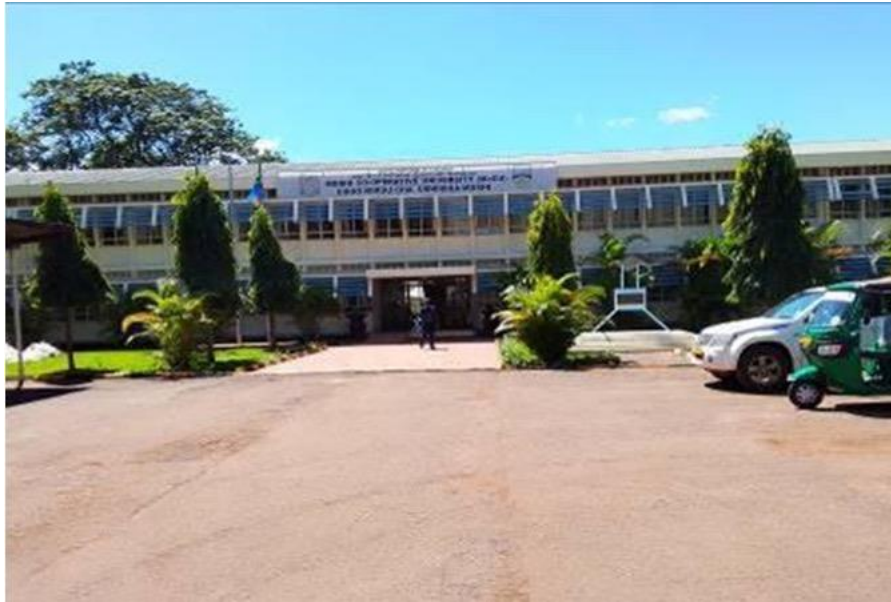
Plate 1: Administration building within MoCU main Campus (Source: Field Visit on 7 th June 2023)
